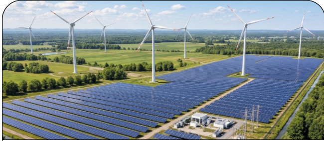
Hybrid Power Plant
