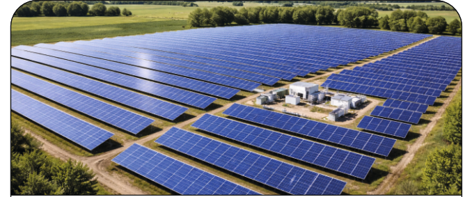
Solar Ground Mount
